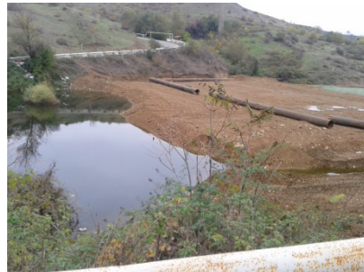
Runoff collector pond at upstream end of dam
