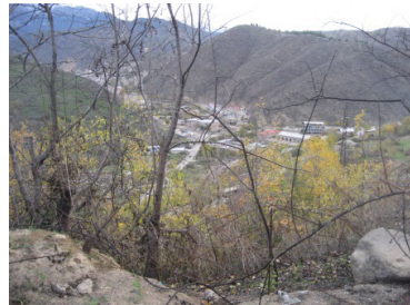
Downstream industrial installations, banks of River Voghji
