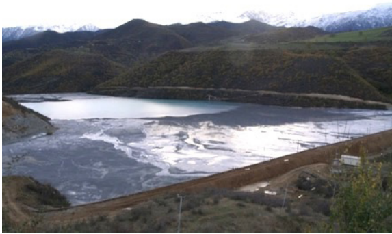
Upstream raise tailings dam with signs of ARD in dam wall (Syunik Province).
