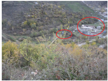
Downstream seepage collector pond area and industrial installation (unoccupied)
