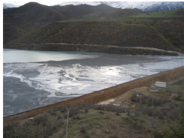
Crest and tailings beach
