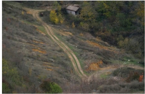
Upstream raise tailings dam with signs of ARD in dam wall (Syunik Province).
