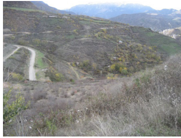
Downstream slope - toe
