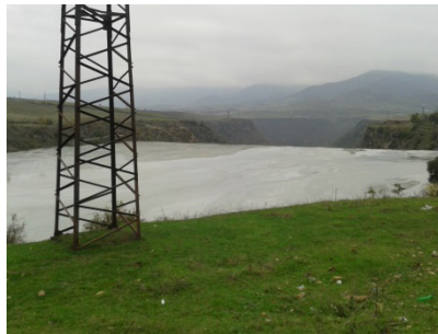
Top surface – view to crest
